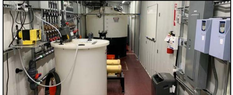
Injection and Extraction System Equipment for a NERT Treatability Study
